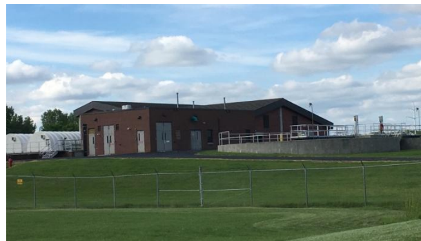
Water Treatment Plant
