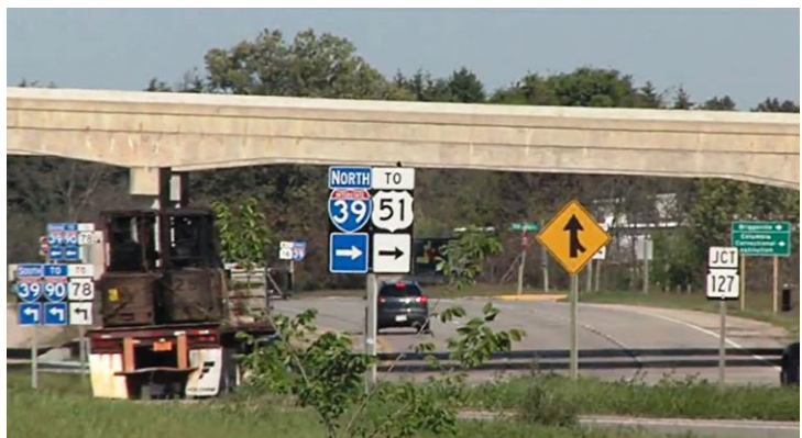
Bridge under Interstate 39
